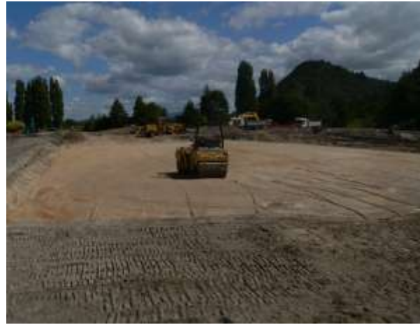
Civil Construction Works at the Station Site
