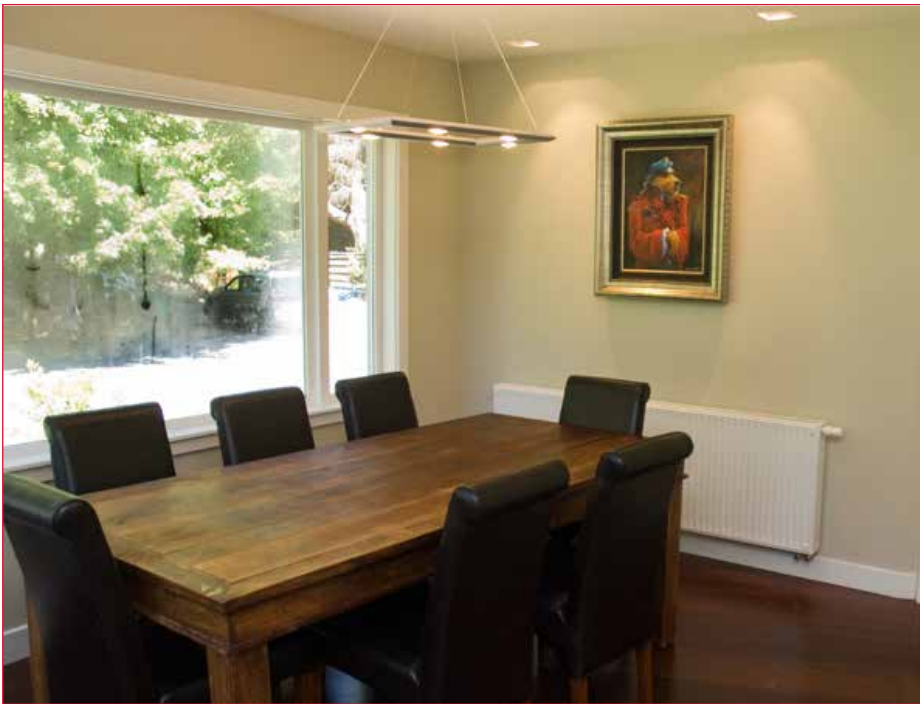
Warm water generated by the heat pump is circulated through radiators.
