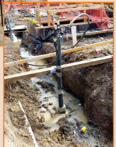
Grouting a ground loop in a borehole
