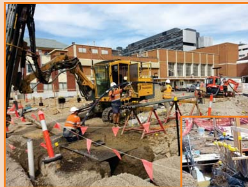
Installing a 50 metre deep ground loop
