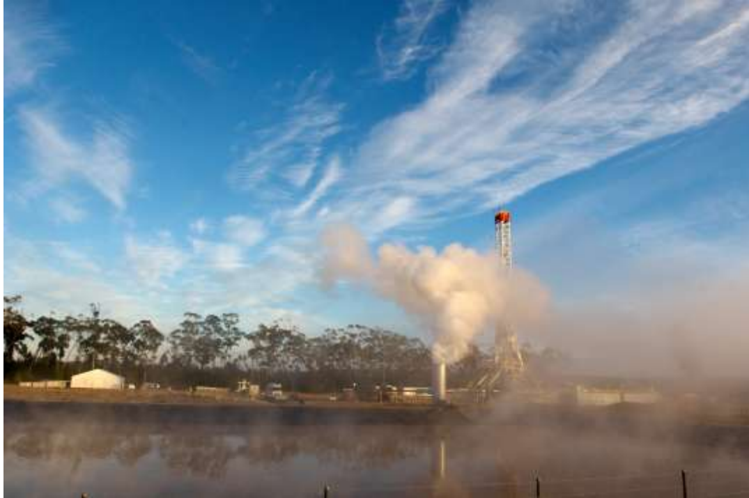
Figure 3: Testing at the Penola project
