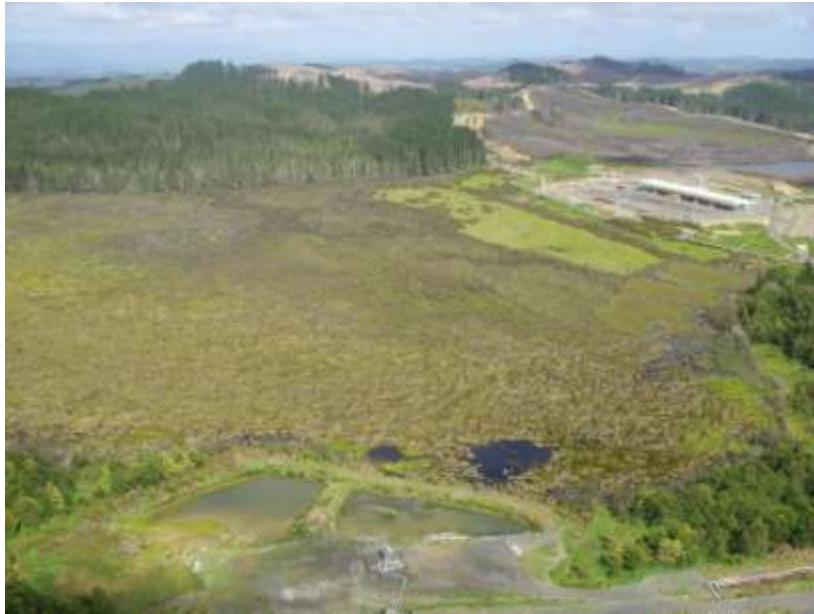
Figure 4: The new Ngawha power station is shown centre right. Extensive bogland in the foreground is protected under QEII open space covenant and the environs are actively managed by the company.
