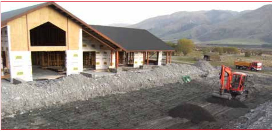
The captor field being installed.
