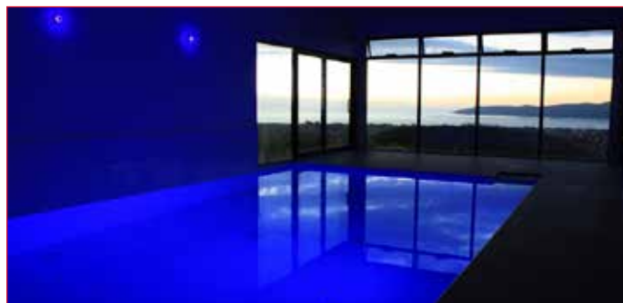
The indoor pool, heated with energy from the earth.
