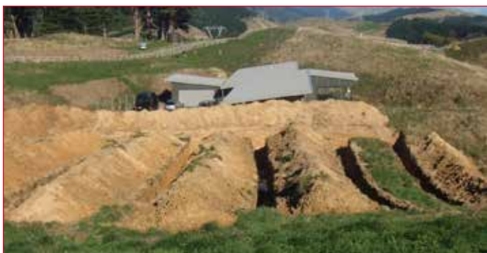
The slinky coils are installed in a network of trenches.
