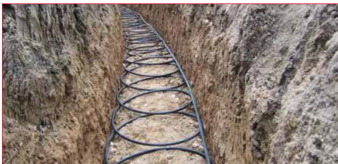
The 'slinky' pipes laid in the trench.
