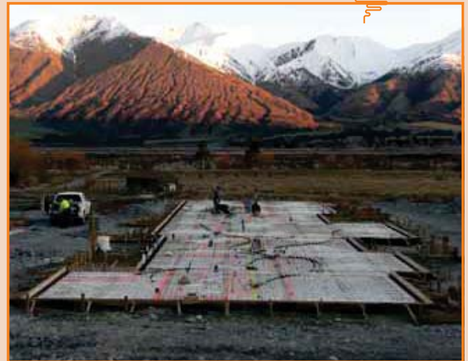
Under floor heating circuits being installed, Manuka Point Lodge, Methven
