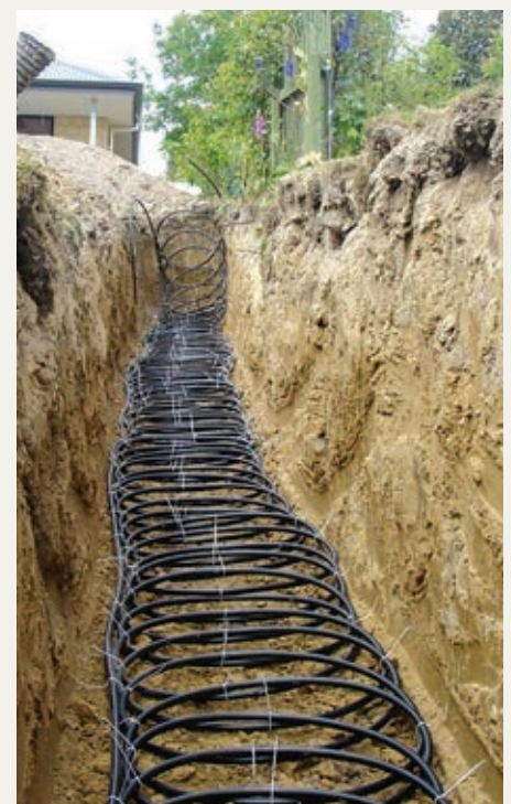
Above: Groundworks for a straight, horizontal closed loop for a geothermal heating installation. Photo: Central Heating NZ Ltd.
